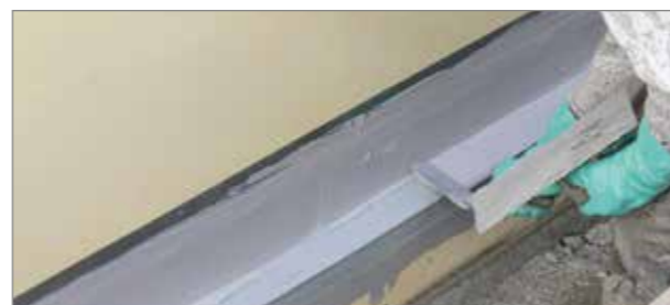
■ 5. Applying the top layer of adhesive
