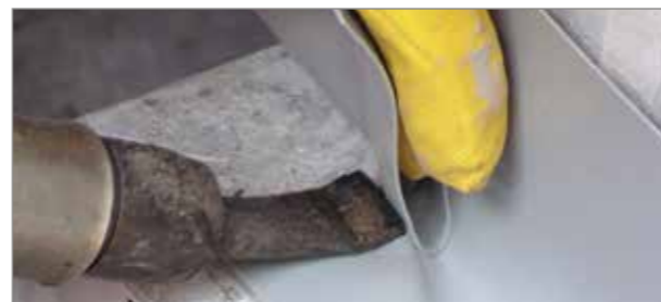
■ 4. Jointing membrane strips by heat welding
