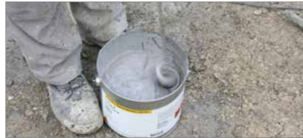
■ 1. Mixing the Sika® Tricoflex® FU 60 system adhesive
