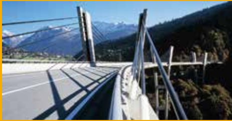
CONCRETE REPAIR AND PROTECTION
