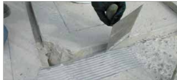
■ 2. Applying the base layer of adhesive
